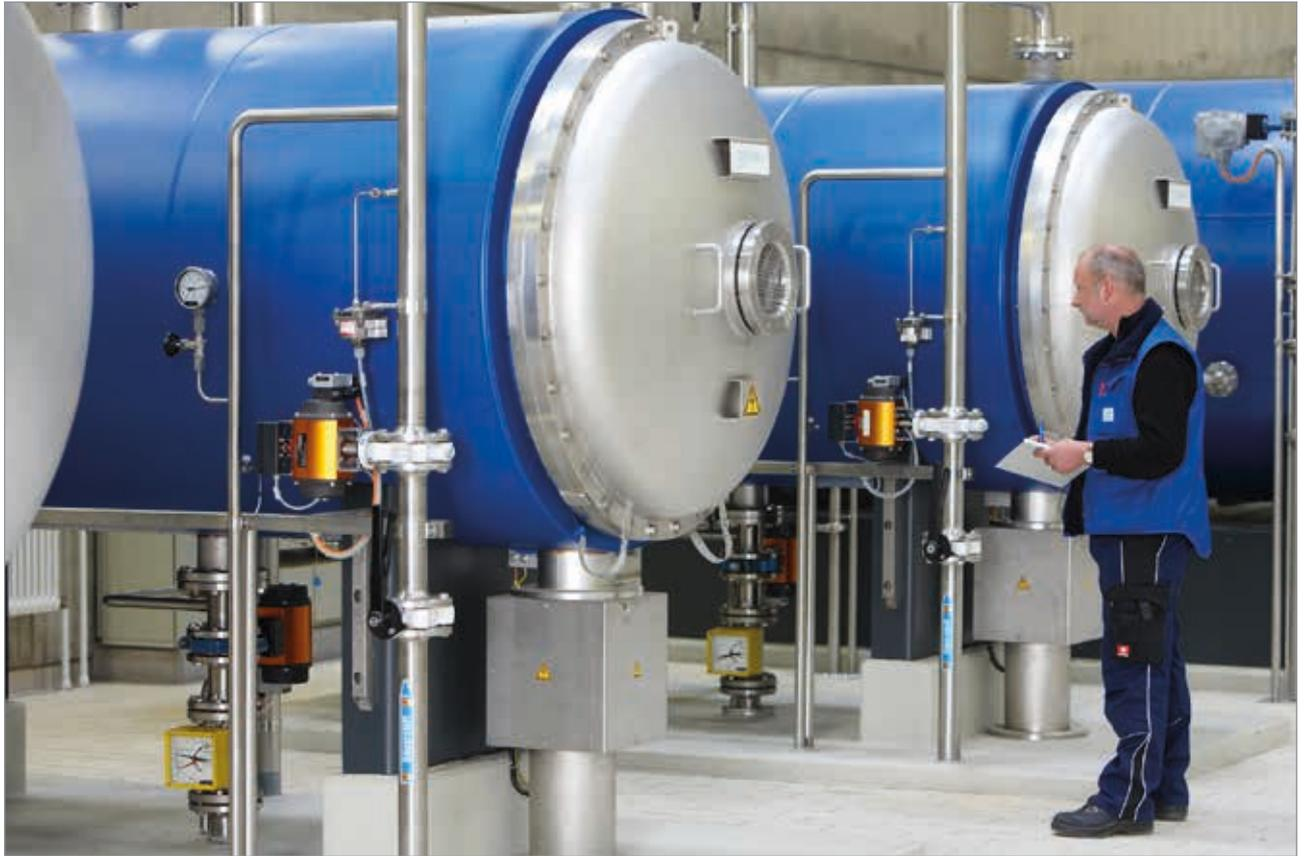
Conversion of oxygen into ozone in so-called tube ozone generators
