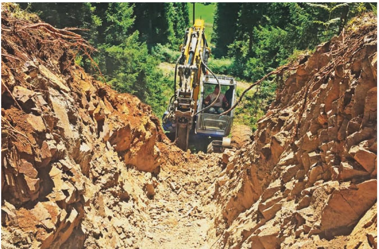
The spider not only dealt with the earth-moving work but it also transported the pipes.
