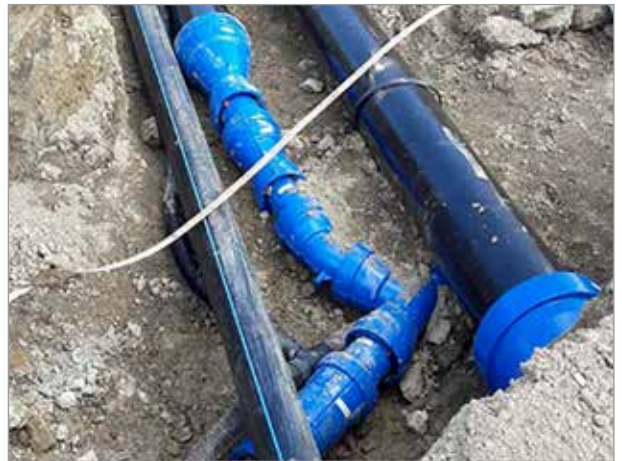
Installation of ductile iron fittings and pipes in tight situations
