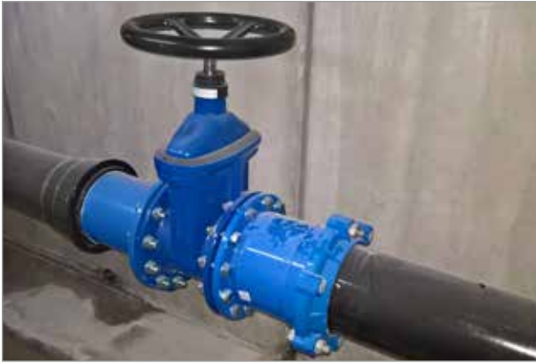
Lateral feed pipeline to the hydrant recesses with ECOFIT fittings.
