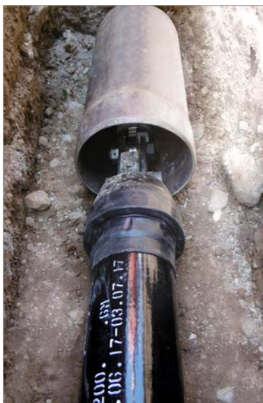
Connecting the traction head to the expansion cone
