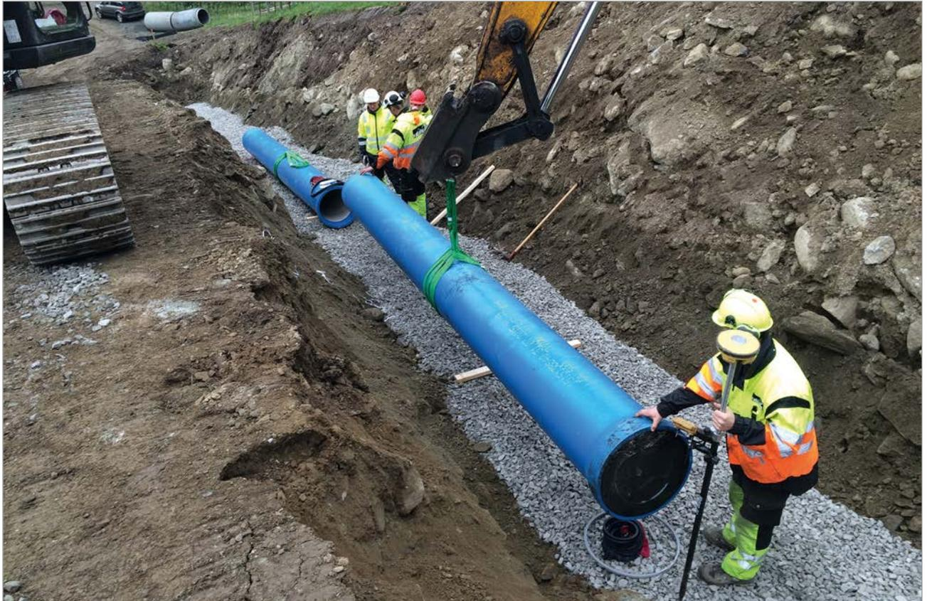
Installation of ductile iron pipes as the turbine pipeline for the Storelvi hydropower station
