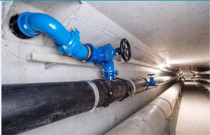
Extinguishing water pipeline in heat-insulated DUCPUR ductile iron pipes with HYDROTIGHT restrained push-in joints, showing a side branch running to the hydrant niches.
