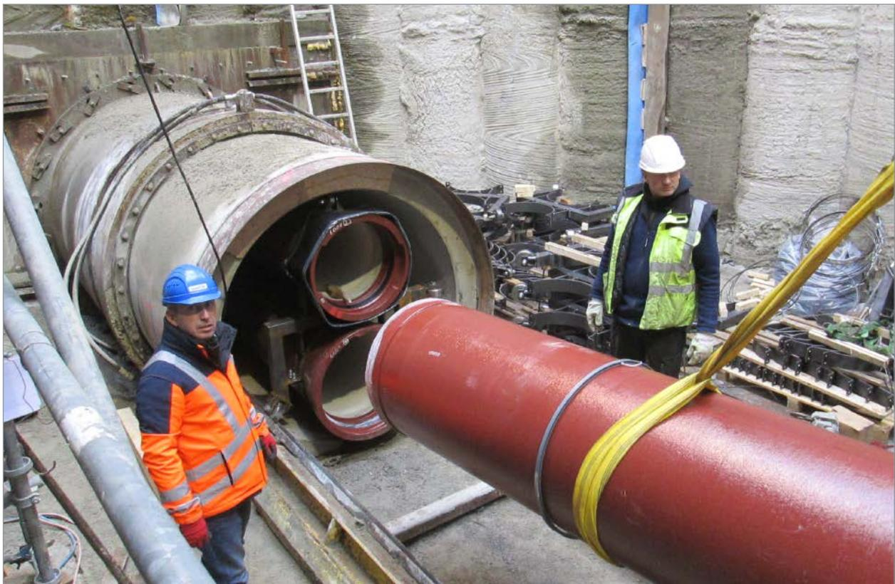
Installation of a DN 600 ductile iron pipe with a BLS® restrained push-in joint
