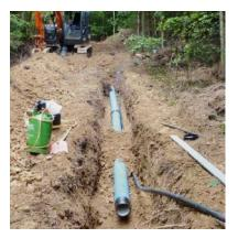
from the construction company carrying out the work. Also, the existing pressure reducing station on Asbacher Straße in Linz am Rhein had to be reconnected and the Sternerbach stream had to be crossed. For the crossing, in addition to the bridge construction, a steel protective casing was installed through which the new pre-insulated water transport line was pulled in. Directly behind the stream crossing the new pipe was connected up to the existing water transport line.
