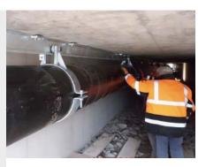
♦ In the context of the construction work a roughly 300 m long DN 300 drinking water pipeline in the Schwarzbach vallev had to be relocated. The water supply association for the district of Aschafftal in Goldbach selected the new route for the drinking water pipeline so that a 160 m long section could be laid using the open trench technique. For this section, DN 300, K 9, PN 10 ductile iron pipes with
