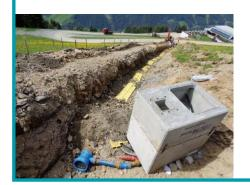
"technical snow". Therefore, in 2014 the Saalbach cableway company decided to construct a new snowmaking system and a new storage reservoir. The Polten storage reservoir has a capacity of 83,700 m³. Ductile iron pipes were used for the snow making pipelines. Back in 2014 around 1.5 km of DN 250, PN 40 ductile iron pipes were installed, with a further 1.5 km following in 2015 in nominal size DN 200, PN 64. The ductile iron pipes with cement mor-
