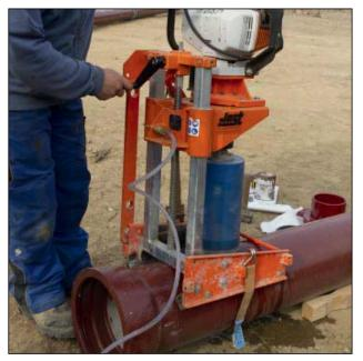
**Fig. 19.30:** Drilling with the core bit
