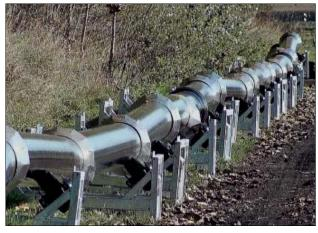
**Figure 22.30:** HDD – elevated pre-assembled pipe string
