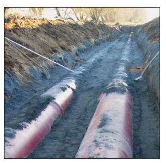
Fig. 9.41: Parallel installation of DN 600 ductile iron pressure wastewater pipelines with BRS<sup>®</sup>/ TYTON SIT PLUS<sup>®</sup> push-in joints
