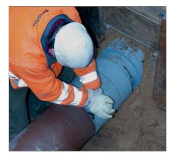
**Figure 22.44:** Coupling for ductile iron pipes
