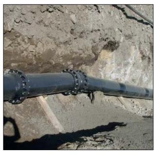
**Fig. 9.45:** A DN 400 turbine pipeline
