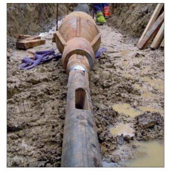
Figure 22.11: Diagram of static burst lining-technique
