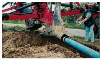
**Figure 22.38:** Plough with upsizing unit
