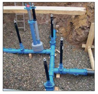
**Fig. 9.44:** Renovation of a gate-valve-equipped pipeline intersection with BAIO<sup>®</sup> restrained joints.
