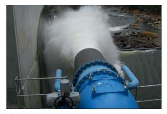
**Fig. 7.6.3:** Plunger valve DN 800, PN 10, with aeration as a bottom outlet valve in the wall of a dam
