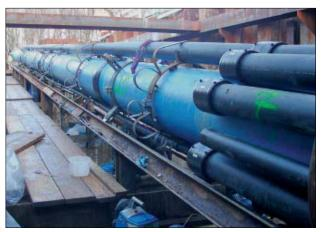
**Figure 22.51:** Sewage pipeline – guided roller brackets
