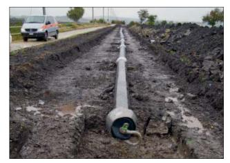
**Figure 22.29:** HDD – pipe string pre-assembled in the trench
