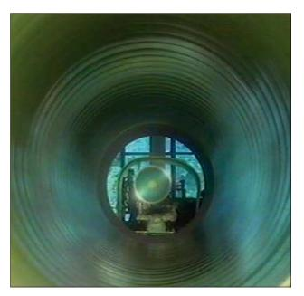
**Fig. 3.28:** Applying the PUR lining using a lance with rotating nozzle
