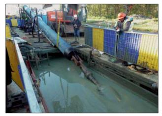
**Figure 22.32:** HDD – individual pipe assembly using an assembly ramp
