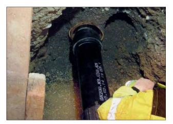
**Figure 22.47:** Relining DN 200 (new) cast iron pipe in an old DN 300 cast iron pipe
