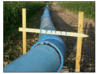
**Fig. 9.34:** Negative angular deflections at a bend – Checking the shift of the bend to the neutral-angle position
