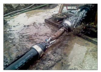
Figure 22.27: Positioning the swivel between reamer and traction head
