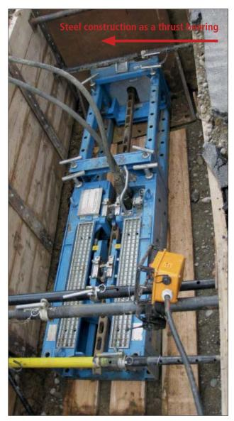
**Figure 22.17:** Traction unit and thrust bearing
