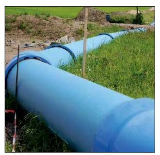
**Fig. 9.43:** A DN 600 ductile iron bypass pipeline with BLS<sup>®</sup> push-in joints
