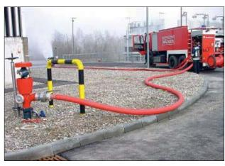
**Fig. 7.8.5-01:** Industrial hydrant for the supply of extinguishing water in industrial plants
