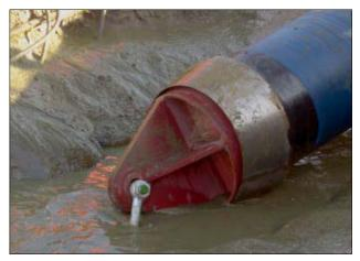
**Figure 22.28:** Traction head with sheet steel cone
