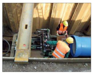
Figure 22.55: Pushing in a pipe
