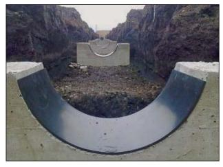
**Fig. 19.47:** Concrete support saddle with neoprene support for ductile iron pipes
