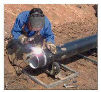
**Fig. 9.5:** A welded bead being applied on the installation site
