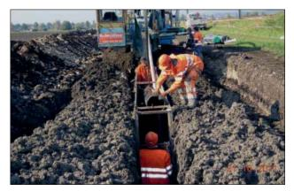
**Figure 22.33:** Cutting in – individual pipe assembly in sliding formwork
