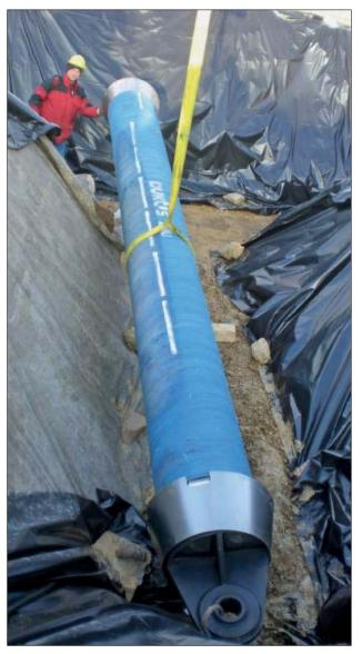
**Figure 22.58:** Pipe with traction head and sheet steel cone
