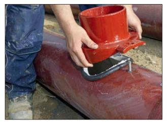
**Fig. 19.32:** Gasket inserted and retaining screws fitted
