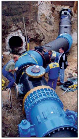
**Fig. 9.42:** Installation of restrained ductile iron bends
