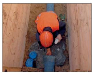
Figure 22.15: Launch and assembly pit
