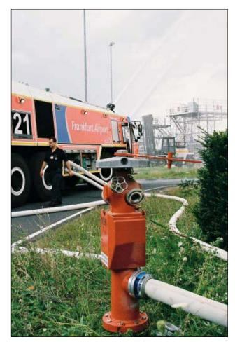
**Fig. 7.8.5-02:** Industrial hydrant for the supply of extinguishing water in industrial plants
