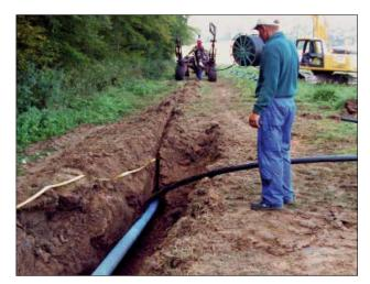
**Figure 22.41:** Pipeline ploughed in
