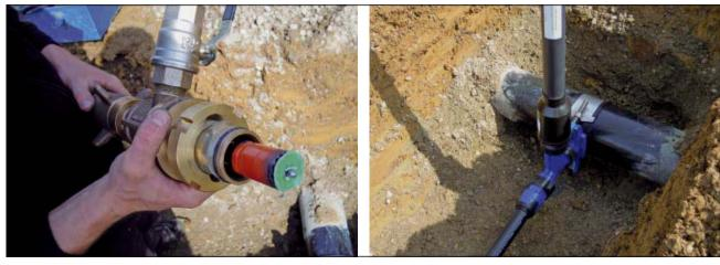
**Fig. 19.34:** Tapping ductile iron pipe using a tapping valve
