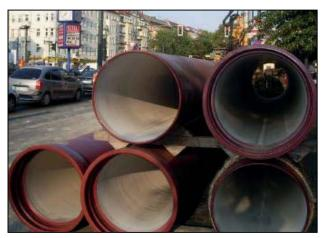
Fig. 8.1: Ductile iron sewer pipes with the TYTON<sup>®</sup> push-in joint
