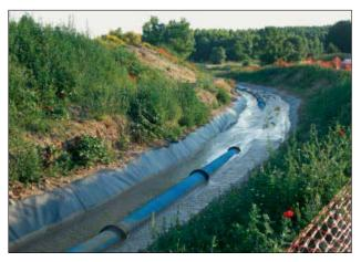
**Figure 22.31:** HDD – pre-assembled pipe string floating in the bentonite suspension
