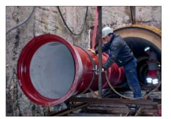
Figure 22.52: Sewage pipeline – assembling the roller brackets
