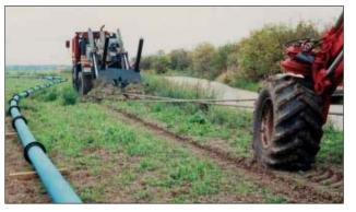
**Figure 22.37:** Steel cable to the towing vehicle
