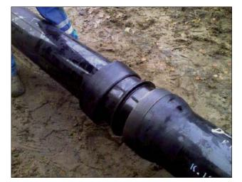
**Figure 22.5:** HYDROTIGHT positive locking push-in joint
