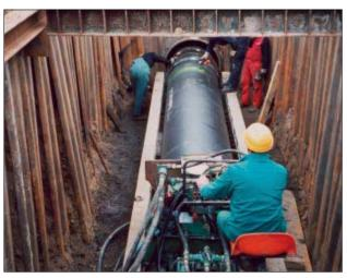
**Figure 22.3:** Pipe relining – pushing in ductile iron pipes
