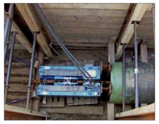
**Figure 22.57:** Traction unit with rods
