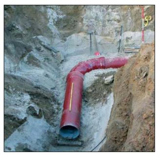
**Fig. 9.40:** DN 700 ductile iron sewer pipes with Novo SIT<sup>®</sup> push-in joints
