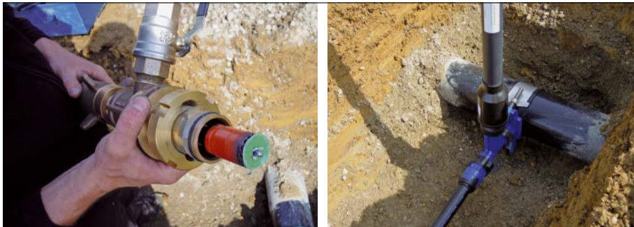
Fig. 19.34: Tapping ductile iron pipe using a tapping valve
