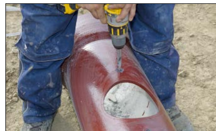
Fig. 19.31: Drilling the holes for retaining screws of the connection branch
