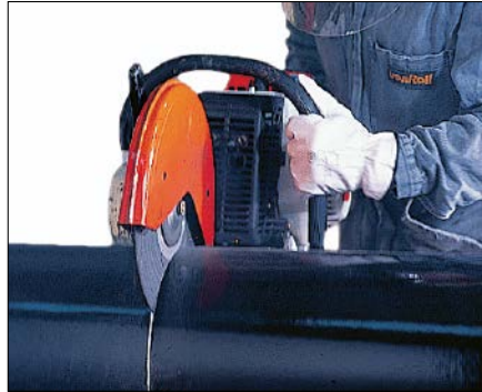
Fig. 19.17: Separation cut on a pipe
