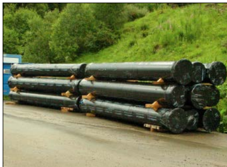
Fig. 19.5: Ductile iron pipes set down on wooden supports
