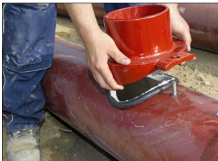
Fig. 19.32: Gasket inserted and retaining screws fitted
