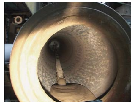
Fig. 15.1: Charging the pipe with cement mortar before the spin centrifuging
