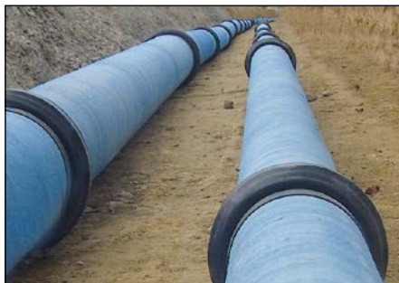
Fig. 14.13: Ductile iron pipes with a cement mortar coating and with rubbers collars to protect the socket joints
