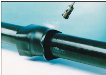
Fig. 14.12: Application of a shrink sleeve
