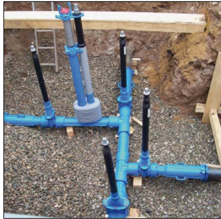
Fig. 9.44: Renovation of a gate-valve-equipped pipeline intersection with BAIO® restrained joints.
