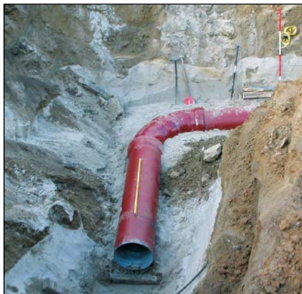
Fig. 9.40: DN 700 ductile iron sewer pipes with Novo SIT® push-in joints
