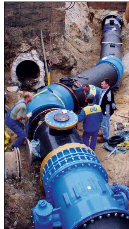
Fig. 9.42: Installation of restrained ductile iron bends
