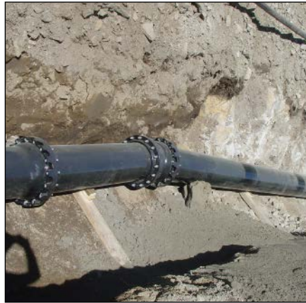
Fig. 9.45: A DN 400 turbine pipeline
