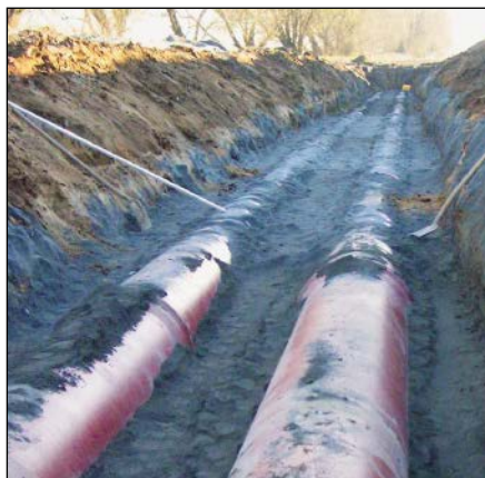
Fig. 9.41: Parallel installation of DN 600 ductile iron pressure wastewater pipelines with BRS®/ TYTON SIT PLUS® push-in joints
