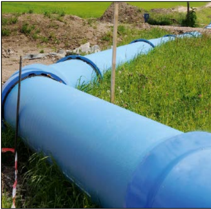
Fig. 9.43: A DN 600 ductile iron bypass pipeline with BLS® push-in joints
