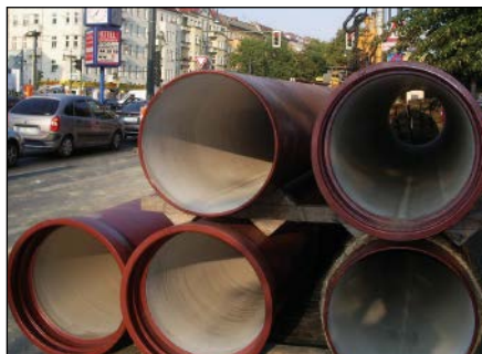
Fig. 8.1: Ductile iron sewer pipes with the TYTON® push-in joint
