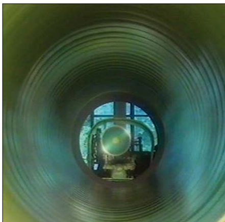
Fig. 3.28: Applying the PUR lining using a lance with rotating nozzle
