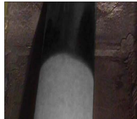
Fig. 3.25: Applying the black PUR coating
