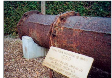
Fig. 1.2: Flanged pipe from the park at the Palace of Versailles
