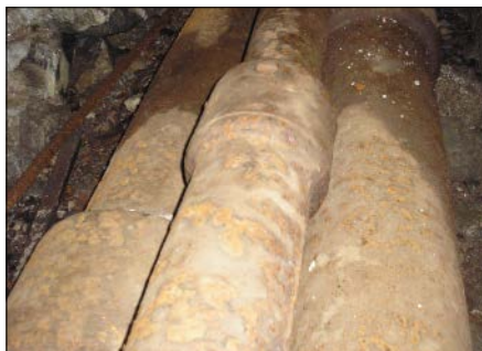
Fig. 1.3: Cast iron pipeline to supply the cascades of the Hercules monument in the Kassel-Wilhelmshöhe castle park with water (UNESCO World Heritage site since June 2013)
